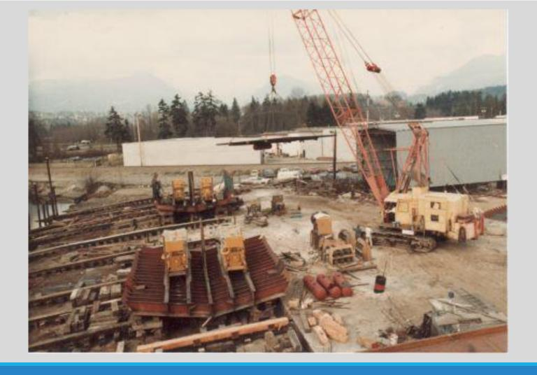
Hull No. 194 and No. 195 – 'Arctic Taglu' and 'Arctic Hooper' Keels Set and Main Engines Installed
